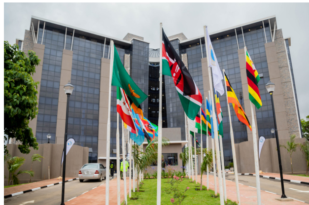
ZEP-RE Office Park in Lusaka
